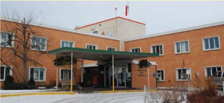
Entrance to Fort St. John Hospital and Wellness Centre
